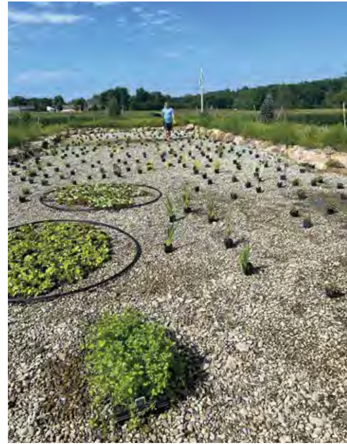
When we planted marginal plants in the bogs, we put the floating hyacinths in anchored hoops so they wouldn't be washed over the falls.
