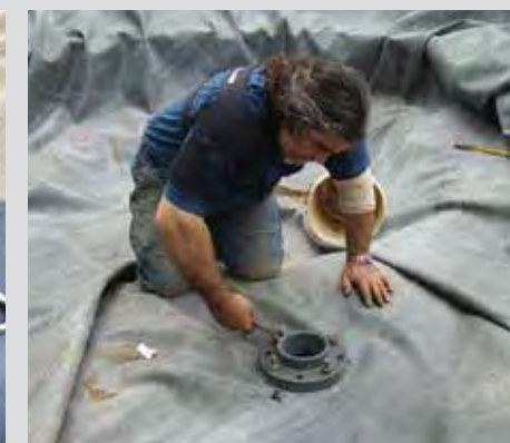
Made with off-the-shelf slip flanges, the only modification is to grind the ridges down flat so the whole flange seals to the liner. We like 5/8" x 3" stainless bolts epoxied into the bottom flange for 4"-8" drains.
