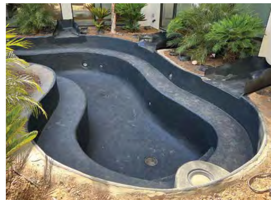
Polyurea is complete, with extra poly on spring returns to be trimmed as necessary.
