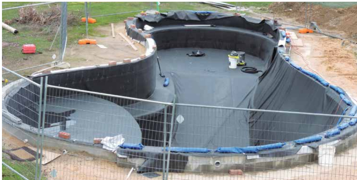
Although EPDM can be custom fit to complex shapes, it pays to not be too ambitious if the budget doesn't allow it. This pool's liner took more than two weeks for two people to install.
