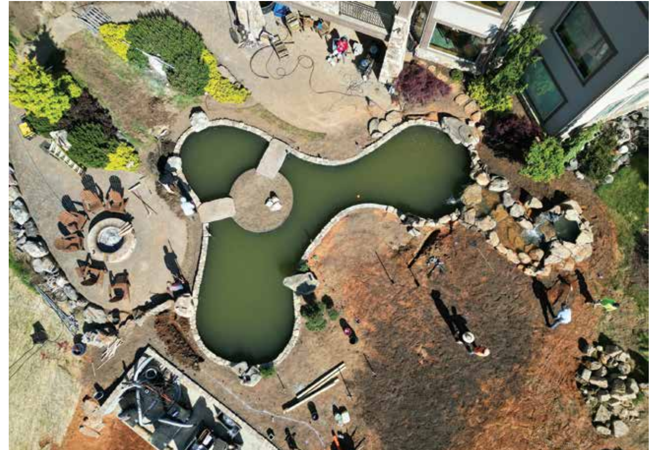
A top-down view of the world's first PolyPond construction process in Roanoke, Virginia, showcasing its unique shape and layout in progress.
