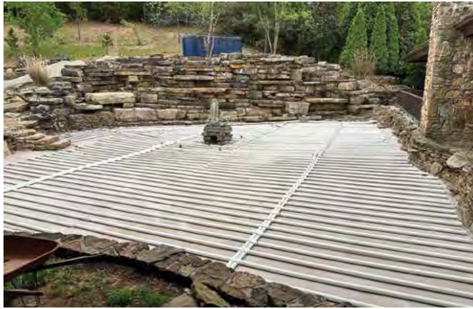
My favorite type of drain is a well plumbed under-gravel filter (UGF) system. This one is 55 x 75 feet and required over 4,000 drilled holes.
