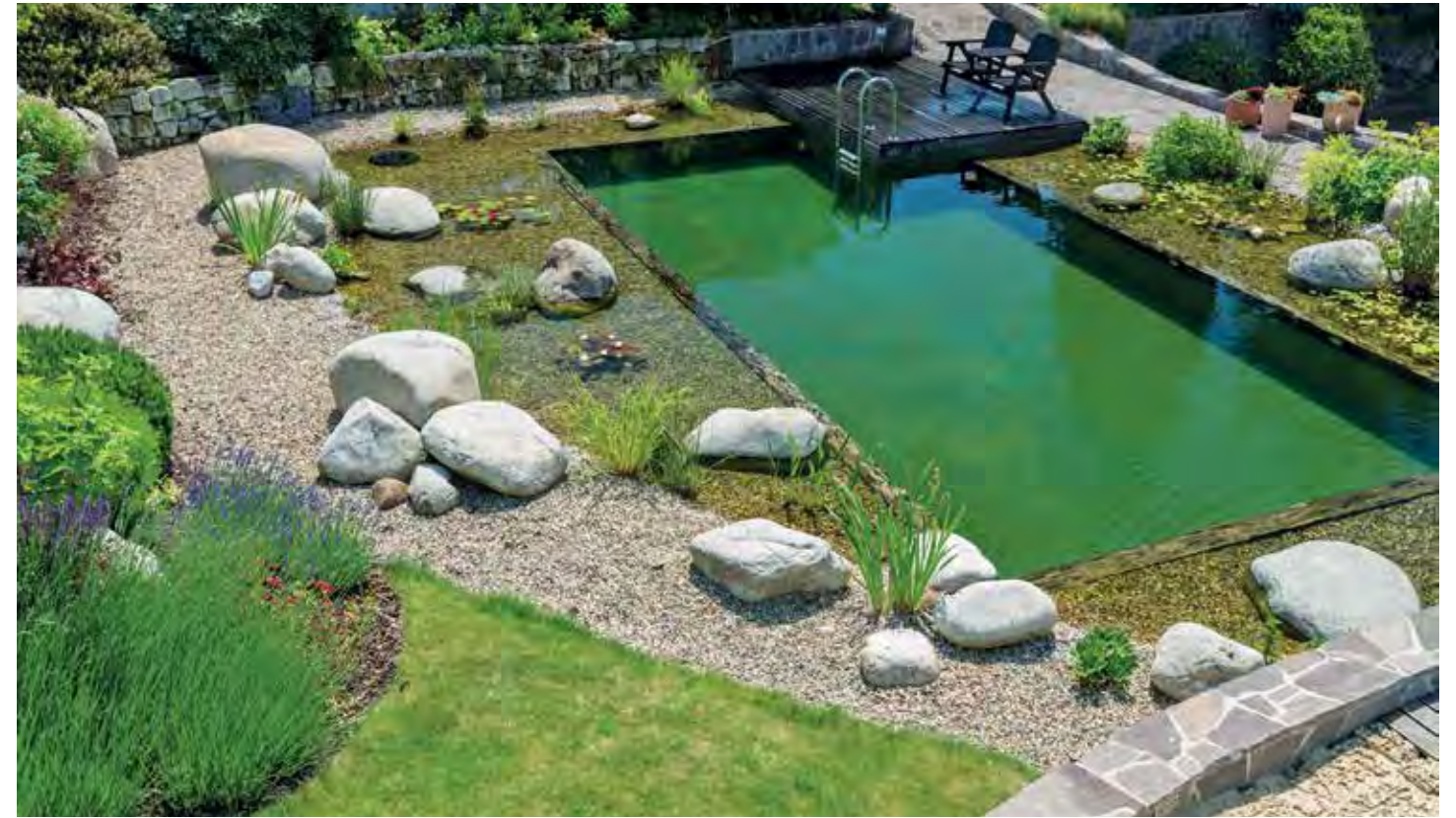
This NSP has a defined swim area, biological filtration in the upflow regeneration (bog) area located around the swim area, and a mechanical filtration system conveniently located under the swim deck at the back of the image.
