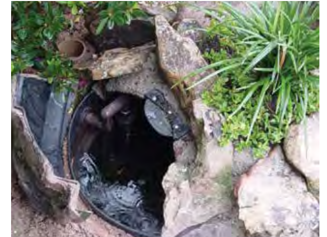
Faux rocks provide the perfect cover for a filtration system.
