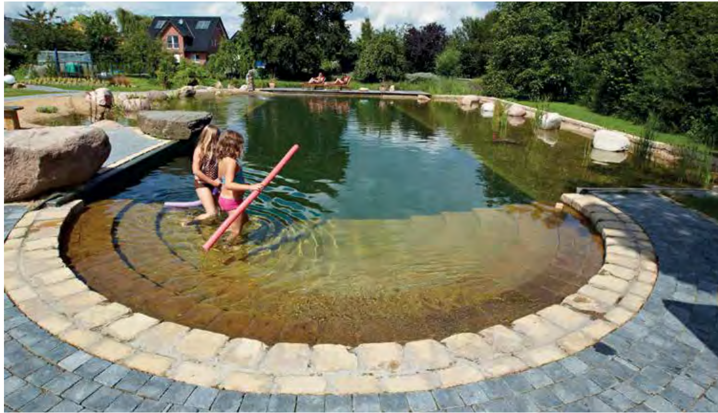
An important part of a well designed NSP is to provide safe ways to enter and leave (ingress and egress) the feature. Additionally, all surfaces in these areas must offer good traction to prevent slips and falls.
