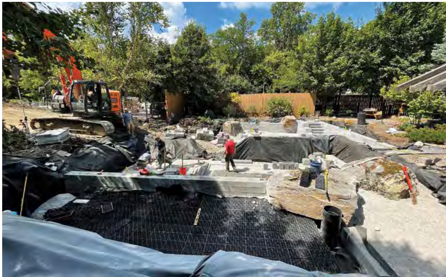
AquaBlox Water Storage Modules create the base of the wetland filtration system for a contemporary recreational pond.
