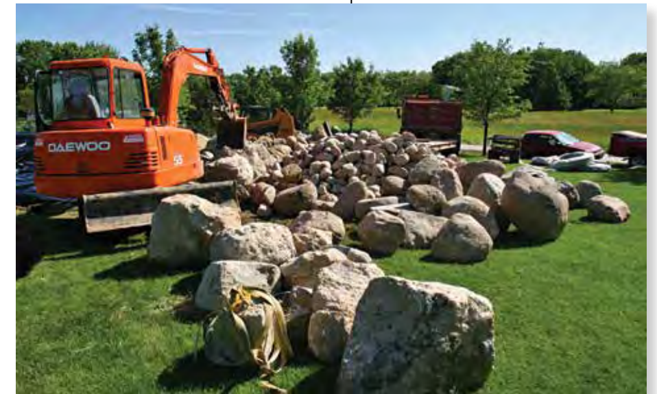
Be sure to plan a staging area for rocks and products when installing a recreational pond.
