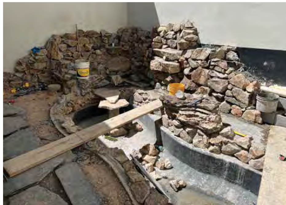
The large boulders (above, left) were the most difficult to place. The equipment area (above) has a sand and gravel filter on a shelf for gravity flow. The rock wall (bottom left) is outfitted with spills and planting pockets.
