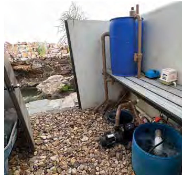
The large boulders (above, left) were the most difficult to place. The equipment area (above) has a sand and gravel filter on a shelf for gravity flow. The rock wall (bottom left) is outfitted with spills and planting pockets.
