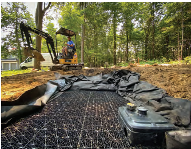
Twelve large Aquascape AquaBlox (left) make up Elaine's 400-gallon reservoir, which is designed to run throughout freezing New England winters. Wide pooling areas slow down the water (right) between the rushing falls and provide ideal drinking spots for some of the birds that Elaine loves.
