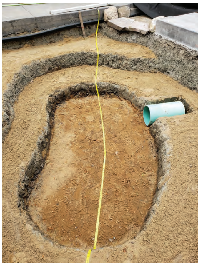
The stamped-concrete pathways (top, left) are under construction before my pond work begins. The pond liner-stream attachment (bottom, left) is detailed relative to the stamped concrete. The 30-inch-deep pond dugout (right) is shown with the sand-bed layer and fish cave PVC pipe.
