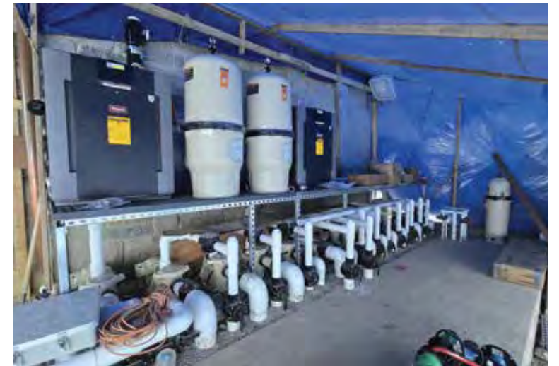
Behind the scenes, an entire wall of pumps, filters and heaters powers the grotto’s massive waterfall system—keeping water clean, moving and ready to enjoy.
