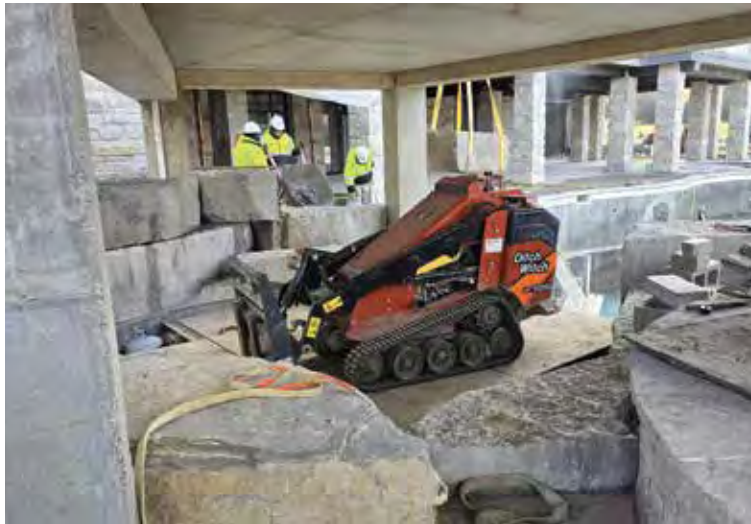
Our mini skid steer rests on a makeshift “road” built over the sunken pool, giving us access to the worksite from the inside. Our crew sets mortar as a crane holds the rock in place.
