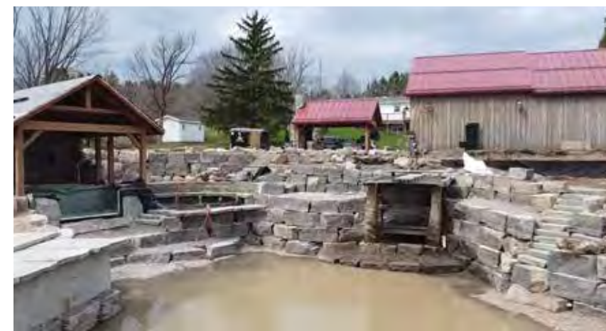
(Top) Phase 1, the architect's final design. - (Center) Phase 2, the pond design sketch by Brent Bivona. - (Bottom) A peek into what lies beneath the surface of the pond. Here you can see the glass viewing window, sitting ledge, stairs and grotto.
