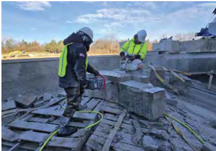
In the frozen winter cold, the team cuts both horizontally and vertically to shape a rock that will cantilever over the pool’s edge.
