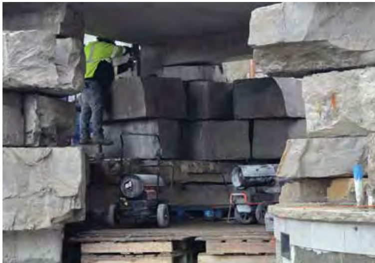
Diesel heaters kept the space warm enough to work through the cold winter, while a pallet-and-plywood platform gave us a safe work area and a path to move our mini skid steer inside the grotto.
