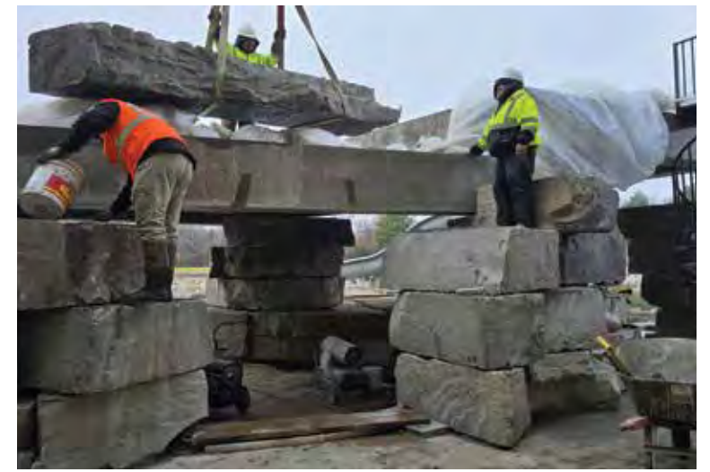
A large span rock is placed on the back side of the grotto. Freezing temperatures often forced the team to dry-stack stones and later take them apart to reset with mortar once conditions improved.
