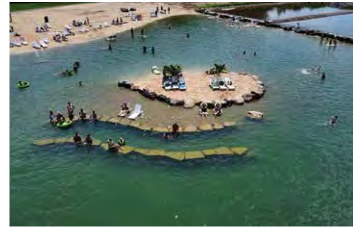
The natural swimming pond features shallow beach entry, a small central island for lounging and natural stonework for sitting and conversation. The stonework also defines the different swimming zones.
