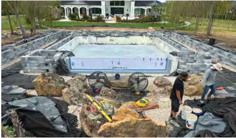
The acrylic viewing window was installed as construction of the block walls was completed and work began on the pond's waterfall features.
