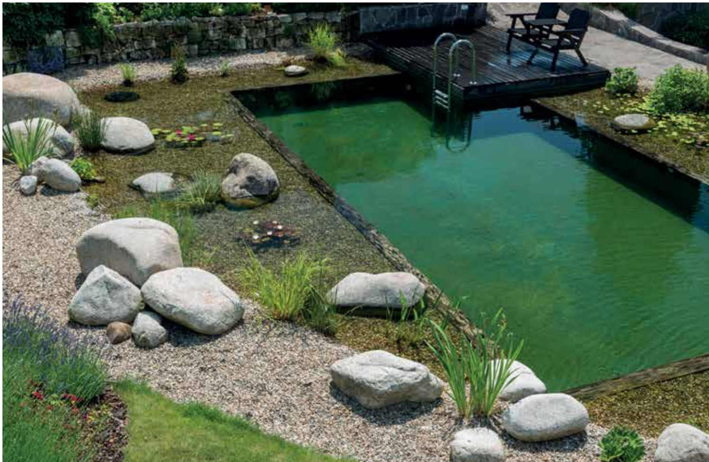
Type 3: Pond is filtered mostly by a planted regeneration zone, but assisted by mechanized filtration.
