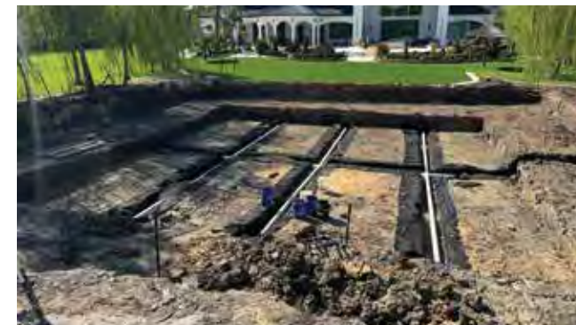
Left: French drain installed beneath the liner. - Right: Liner completed and AquaBlox matrix installed, forming the underground reservoir system.
