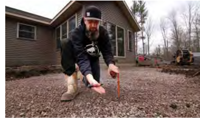
Dan, laying out the footprint for his a patio project.
