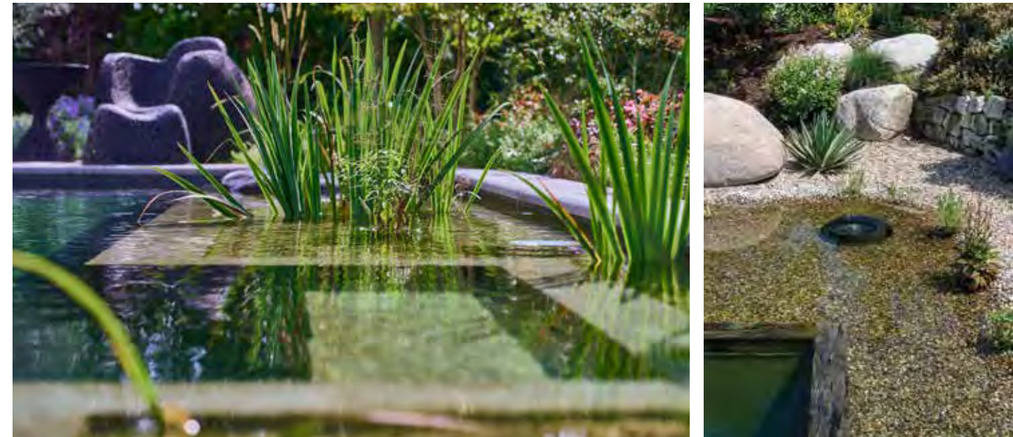
Left: Plantings in the Regeneration zones remove nitrates from the water. - Right: In-gravel skimmers, like the ProfiSkin, clear debris in the shallow Regeneration zones
