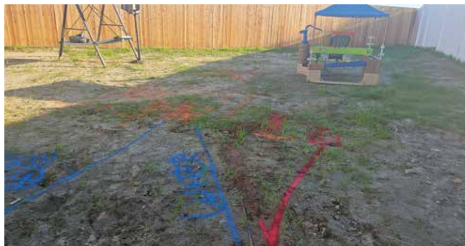
Marking out the future pond and sensory water feature.
