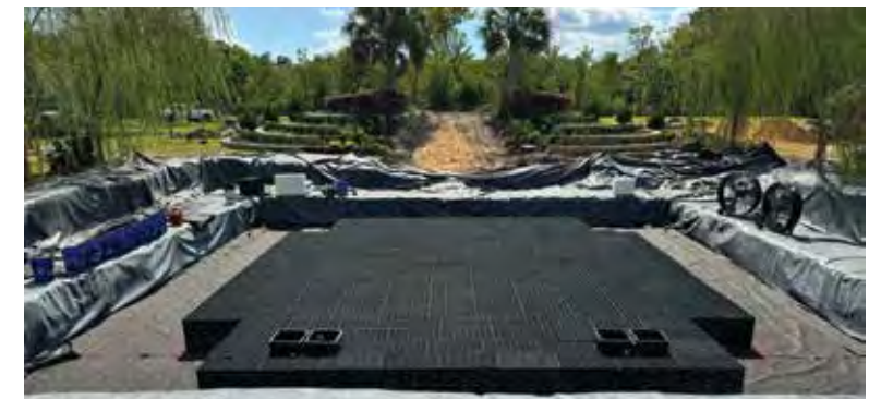
Left: French drain installed beneath the liner. - Right: Liner completed and AquaBlox matrix installed, forming the underground reservoir system.
